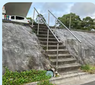
Stairs very steep, steps narrow and have no contrast markings, handrail does not go to the bottom of the staircase. WM
